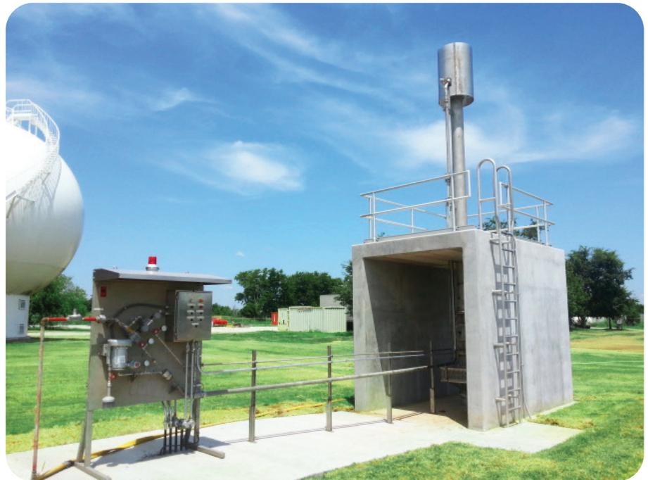
The electronics package controls automatic pilot ignition and monitoring. During the ignition cycle, pilot gas is directed to the flame retention nozzle. Pilot gas is also directed to the venturi where air is inspired. The air/ gas mixture is ignited at the venturi outlet. The ignition generates a flame front which travels through the continuous flame line and exits the continuous flame nozzle at the burner tip. Gas flowing in the flame retention nozzle is ignited by this flame front.
